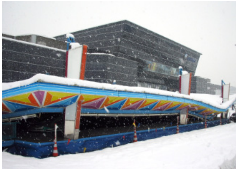
Slika 25. Pod težo snega je klonila streha nad poligonom z avtomobilčki Figure 25. Under heavy fresh snow roof above car playfield broke down
