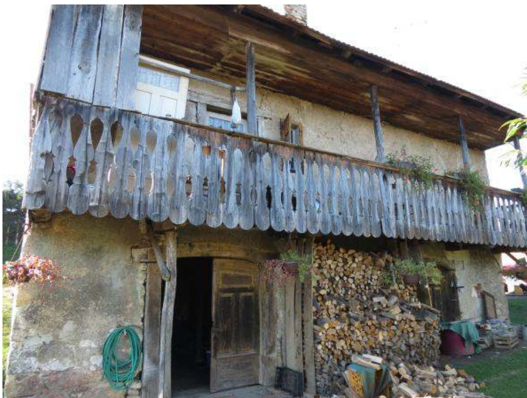
Slika 2. Starejša stanovanjska hiša v vasi Stojanski Vrh, kjer je bil obseg poškodb največji (Starost: 150–200 let, material: zidovi: neobdelan kamen, slaba malta, stropi: leseni, opomba: nepovezano zidovje) (foto: Matjaž Godec) Figure 2. Old residential building in the village Stojanski Vrh, where the damage was the biggest. The house is 150–200 years old, made of rubble stone, weak plaster, wooden floors, external walls not connected (Photo: Matjaž Godec).
