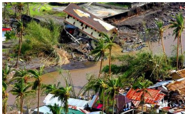
Slika 15. Posledice tajfuna Durian (vir: www.smh.com.au) Figure 15. Typhoon Durian caused a major damage (source: www.smh.com.au)
