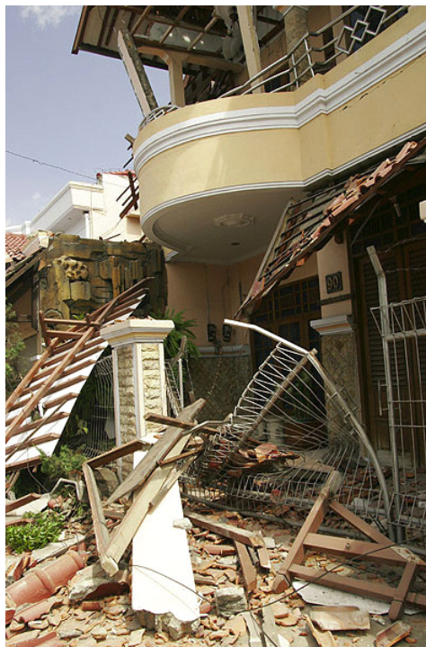
Slika 6. Obsežne poškodbe zgradb v Yogyakarta, Java Figure 6. Extensive building damage in Yogyakarta, Java
